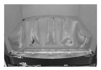
b) Position the two halves of the front ceramic (L/H & R/H) on the locating channel in the front ceramic, ensuring it is located onto the lip on the burner front ceramic support. (See fig. 4 below)
